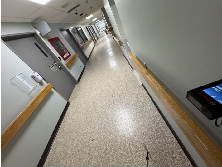
CORRIDOR 01 NEAR SOILED UTILITY (K2E 32) PATCH AND REPAIR DAMAGED FLOORING AT IDENTIFIED LOCATION AND UP TO 10 LOCATIONS OF SIMILAR SIZE AND DAMAGE LEVEL WITHIN AREA. EXACT AREAS TO BE IDENTIFIED DURING CONSTRUCTION.
